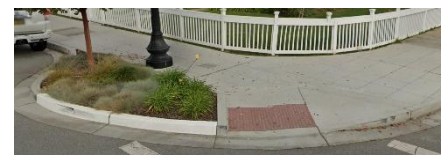
East Side Connect (Old County Road, San Carlos) Bulb-out with nominal ramp slope and adjacent planter
